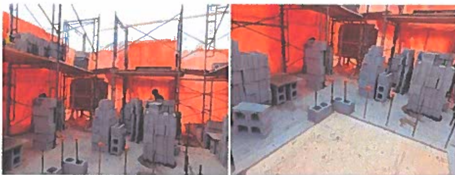
Concrete block being laid up to form the elevator hoist way
