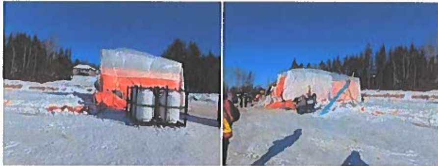
Protective enclosures at stairwells and elevator hoist way provide heat and weather protection to lay concrete block
